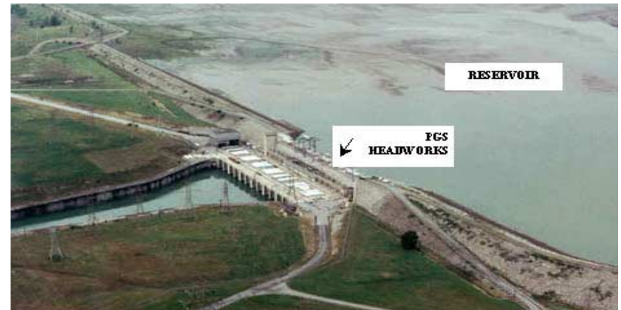
Pump Generating Station
