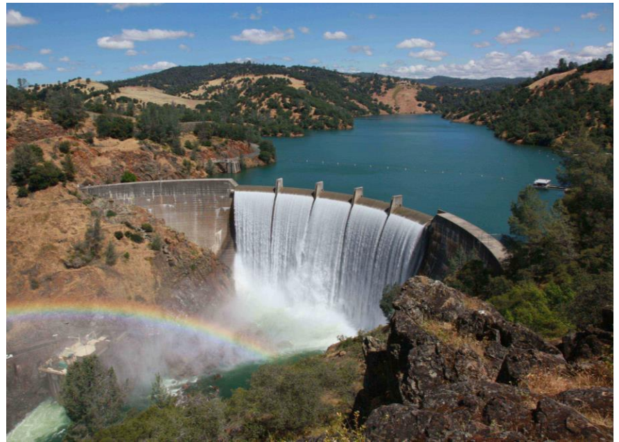
Engelbright dam, Yuba River. US Army Corp
